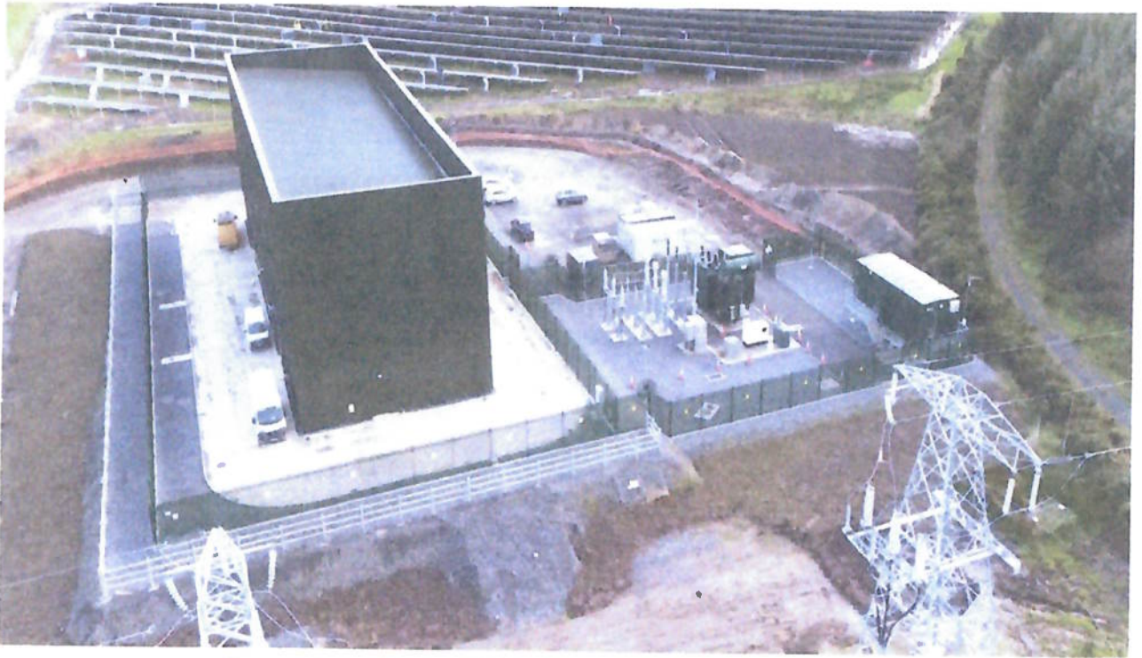
Figure 2-1: Typical 110kV GIS Station Layout (Source: H&MV)
